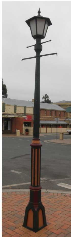
Junee Lamp post Pattern using 17A base and Junee tapered Fluted shaft
