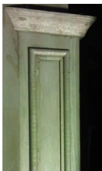
Square Impost with cap and bead trim 110 x 110 mm Impost section. Custom made
